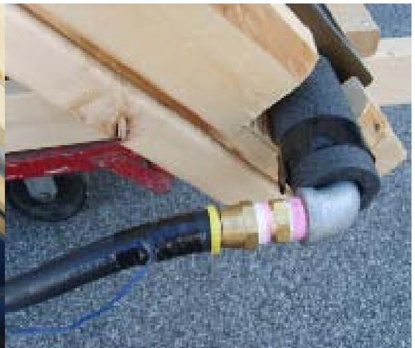
Figure 5: Thermocouple in the hose (solar collector inlet)
