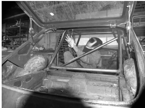
Figure 4 – The student designed roll cage being installed in the IUPUI Engineering Technology racecar.
