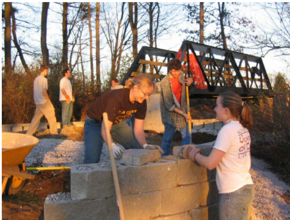
Figure 5: Placing Masonry Blocks for West Ramp (November 2004)
