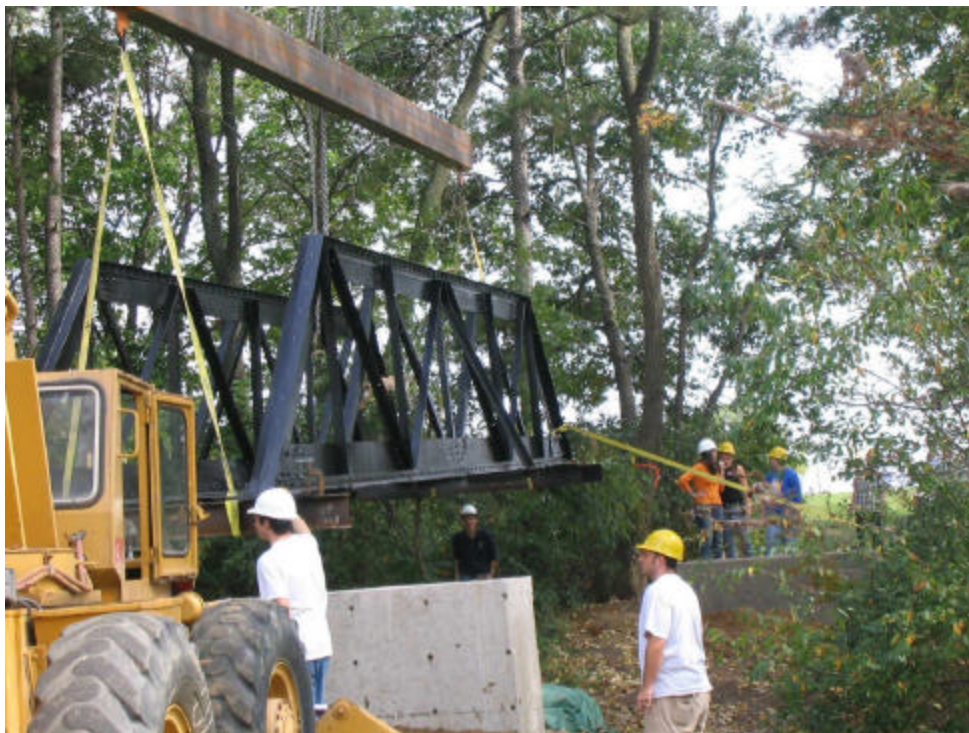
Figure 4: Moving the Bridge Into Place on Abutments (September 2004)
