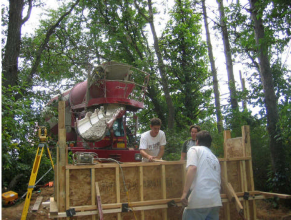
Figure 3: Casting the West Abutment (August 2004)
